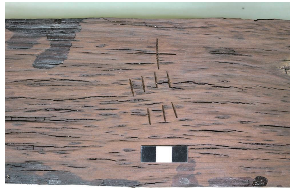
図12 部材に印された文字の一例 (天蓋梁より) Fig.12 Example of Inscription on Wooden Pieces (from a Timber of Canopy)
